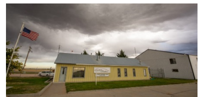
Hayes Aviation, FBO/Terminal Building
