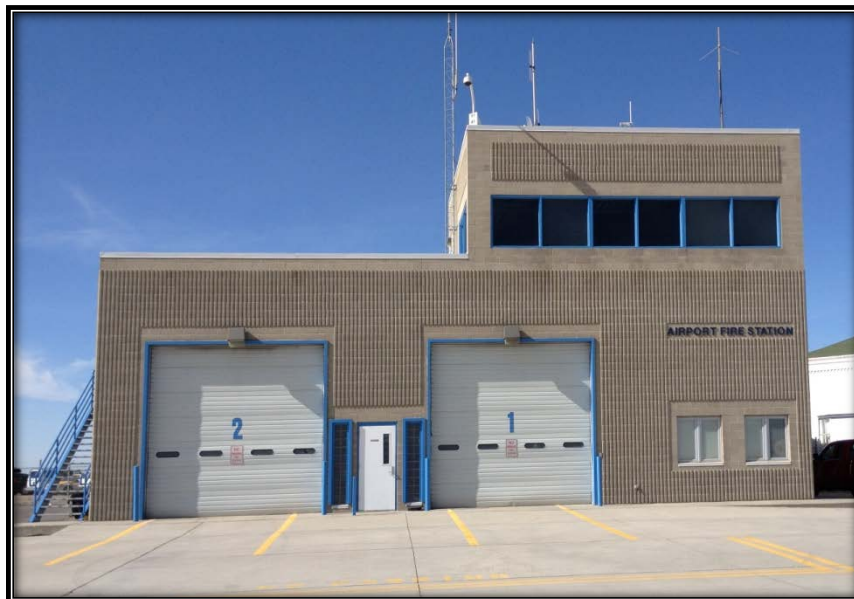
FIGURE 2-10 - RKS'S ARFF STATION
