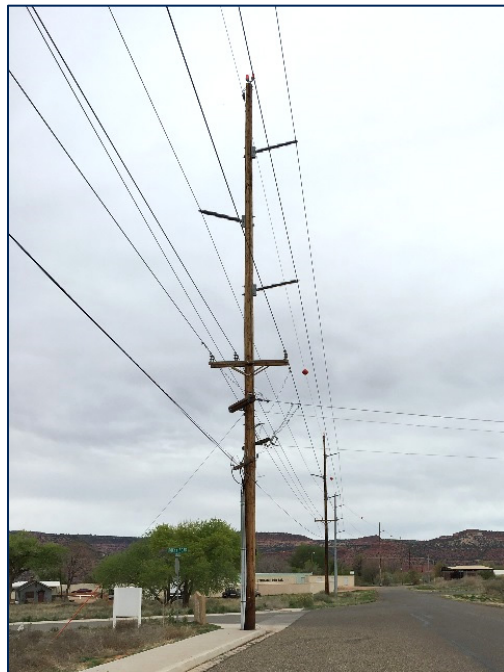
FIGURE 4-6 – UTILITY POLES AND OBSTRUCTION LIGHTS NORTH OF KNB
