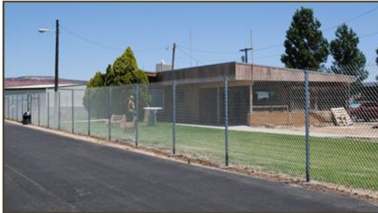
FIGURE 2-9 – EXISTING KNB TERMINAL BUILDING
