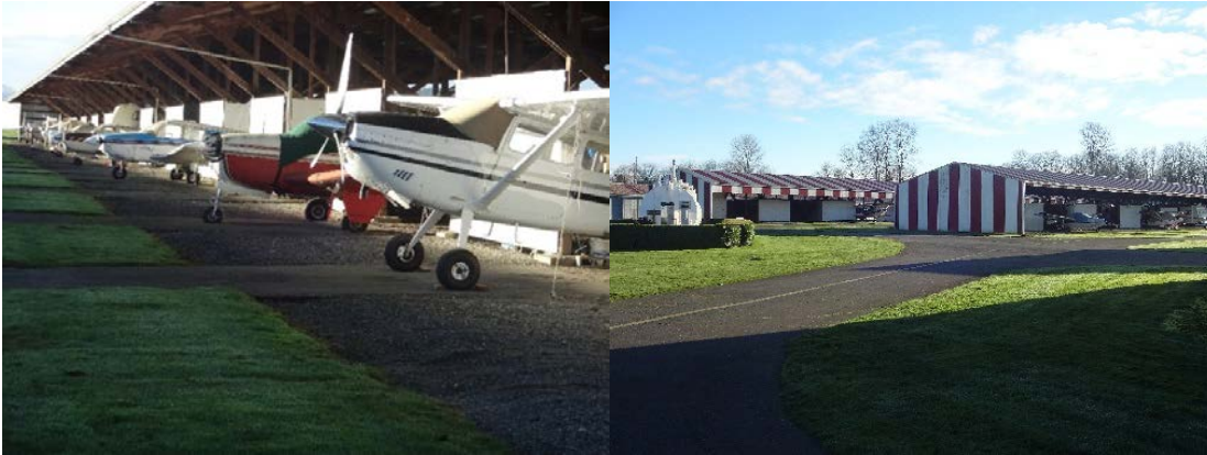
FIGURE 2-12 – S43 SHADE HANGARS
