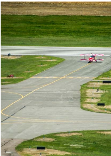
Taxiway A9 at FTG
