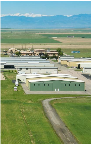
Hangar Buildings at FTG
