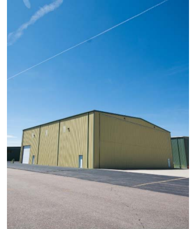
Hangar Buildings at FTG
