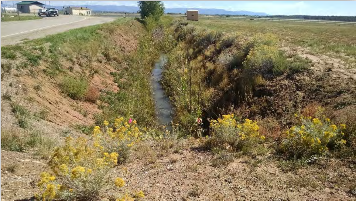
Photograph 14. Looking upstream at the CR 309a roadside drainage conveying irrigation return flows to the Florida River valley floor.
