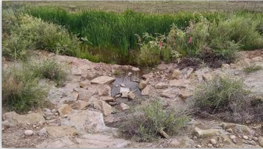
Photograph 5. View looking southeast from airport storm drain into Wetland F.
