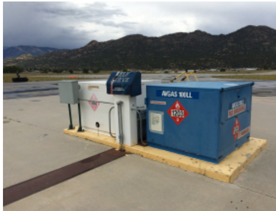
FIGURE 2-12 – SELF-SERVICE FUELING FACILITY
