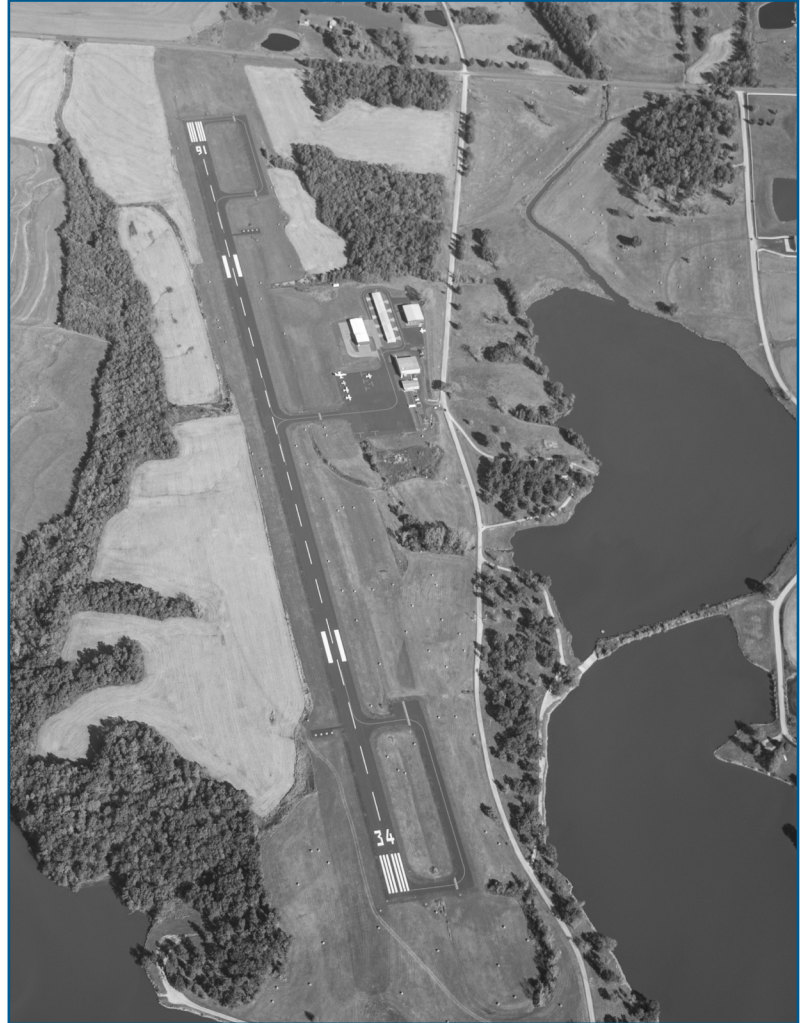
EXISTING AIRPORT FACILITIES FOR HIGGINSVILLE INDUSTRIAL MUNICIPAL AIRPORT
