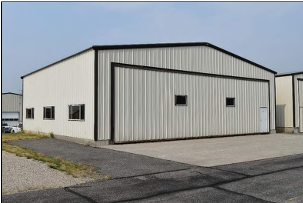
Photograph 36. View of FN-30, facing west (North Wind, August 2020).
