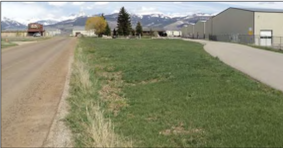
Figure 7. IMG_DSC03241. View east of project area, Driggs-Reed Memorial Airport.
