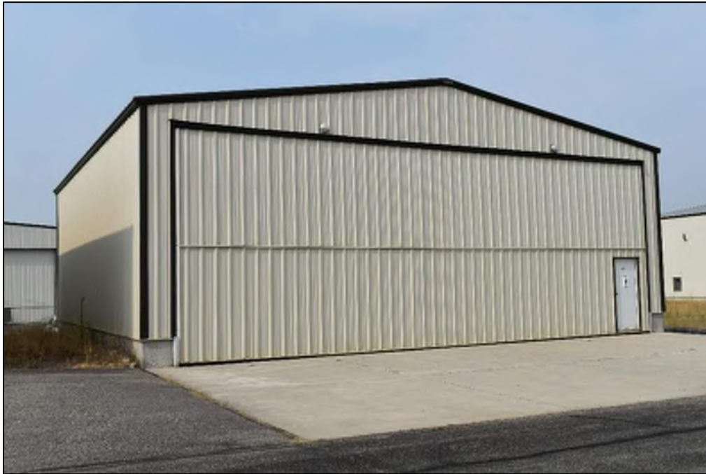
Photograph 33. View of FN-27, facing west (North Wind, August 2020).
