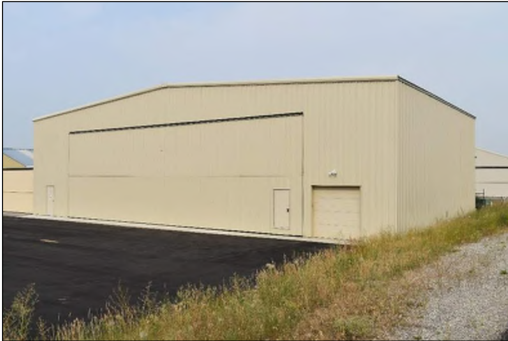
Photograph 15. View of FN-9, facing west (North Wind, August 2020).
