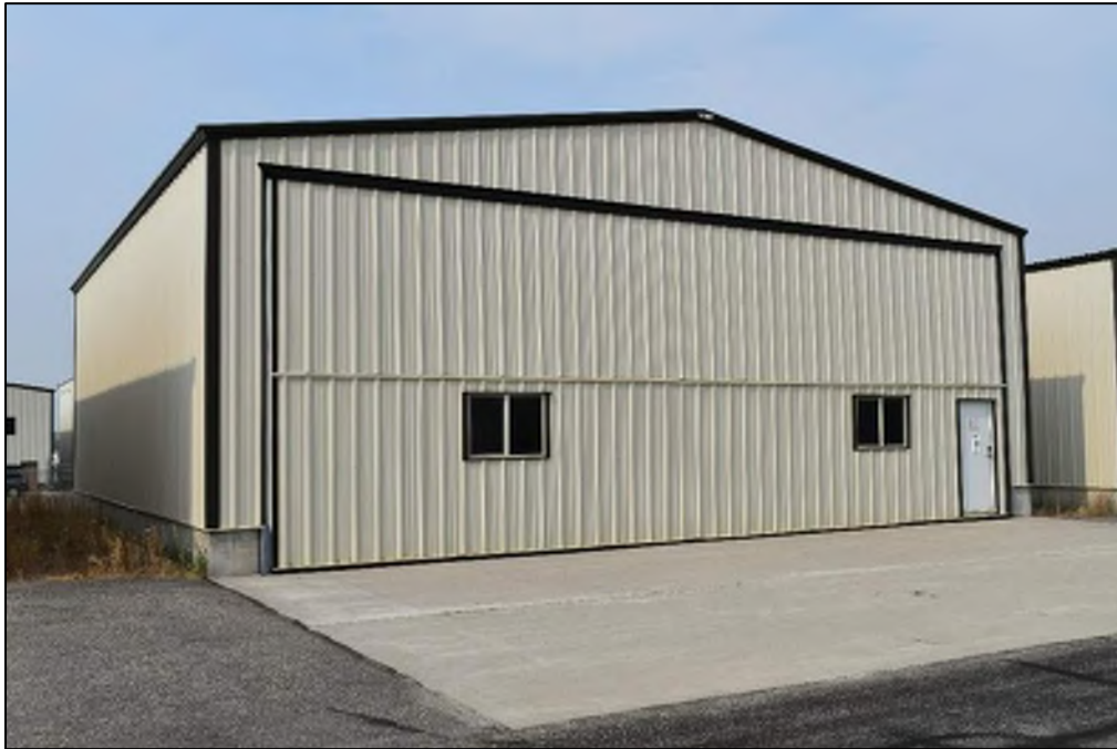
Photograph 35. View of FN-29, facing west (North Wind, August 2020).
