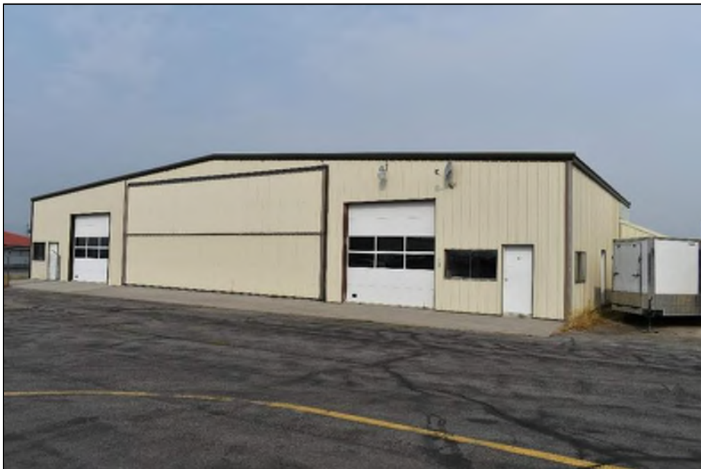
Photograph 24. View of FN-18, facing west (North Wind, August 2020).
