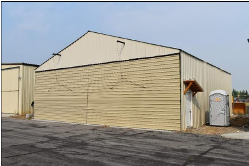
Photograph 26. View of FN-20, facing west (North Wind, August 2020).
