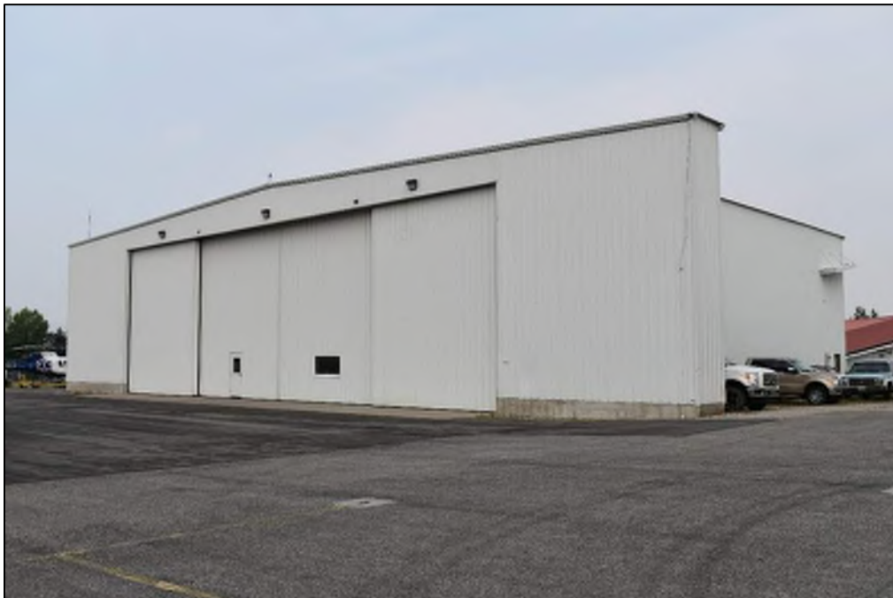
Photograph 8. View of FN-2, facing west (North Wind, August 2020).
