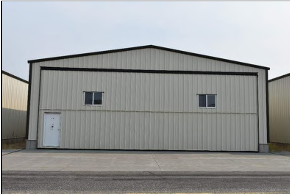
Photograph 39. View of FN-33, facing northeast (North Wind, August 2020).
