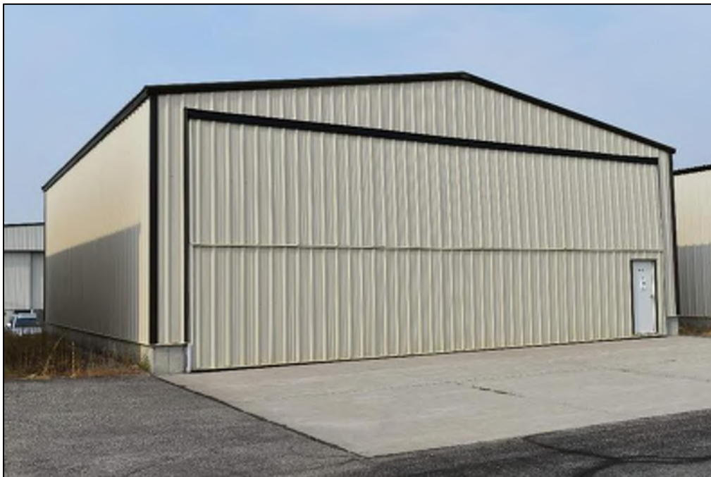
Photograph 34. View of FN-28, facing west (North Wind, August 2020).
