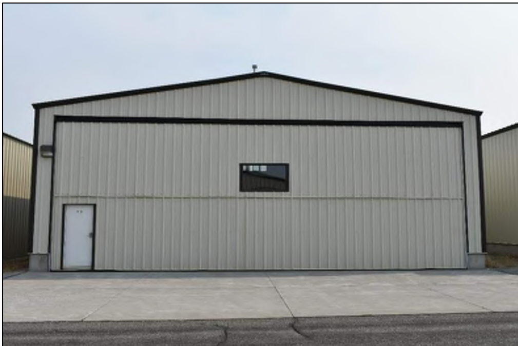
Photograph 38. View of FN-32, facing northeast (North Wind, August 2020).
