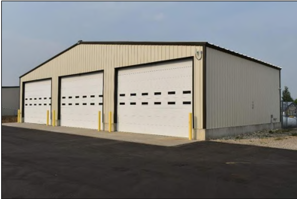
Photograph 43. View of SRE Building (FN-37), facing southwest (North Wind, August 2020).
