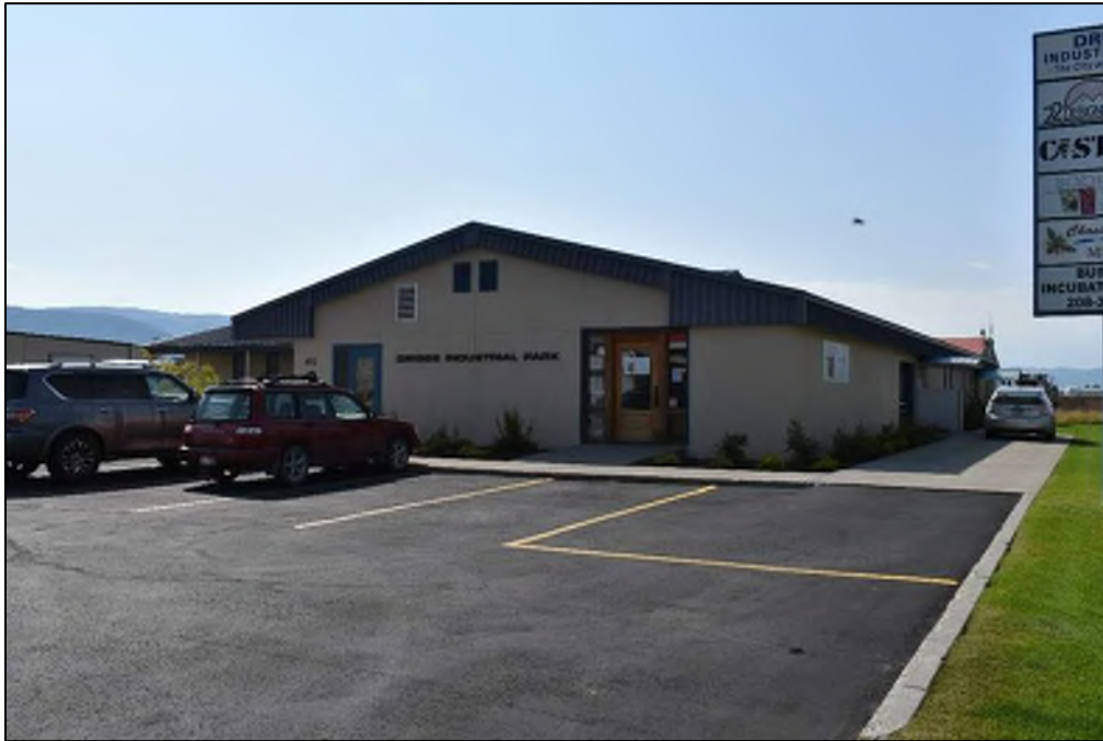
Photograph 45. View of Driggs Industrial Park (FN-39), facing southeast (North Wind, August 2020).
