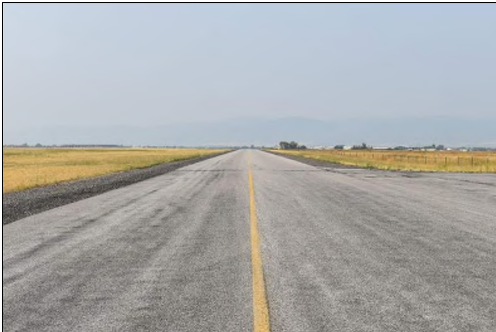
Photograph 42. View of taxiway (FN-36), facing southwest (North Wind, August 2020).
