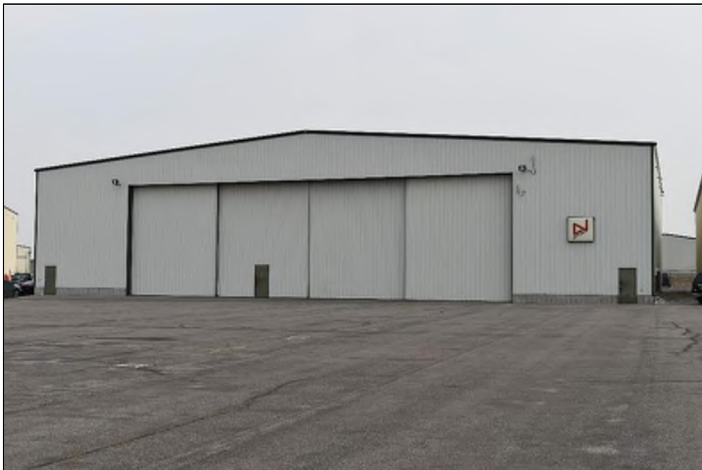
Photograph 32. View of FN-26, facing northeast (North Wind, August 2020).
